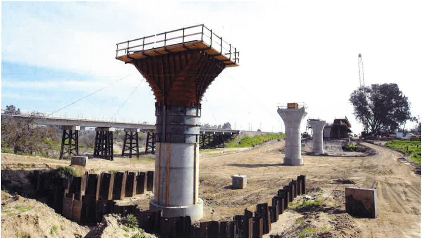
The supports for a 1,600-foot viaduct to carry high-speed trains across the Fresno River are seen under construction near Madera, Calif. (Rich Pedroncelli / Associated Press)
